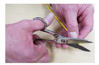
If ribbon fibers are grouped by binder yarn, undo one group at a time as ribbon fibers are inserted into the furcation tubes. If present, trim binder yarn to expose 1/2 inch (13 mm) or less.
