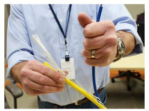
Remove the cable sheath, strength members, tape liner(s), and ripcord(s) at the ring cut, leaving just the central tube.
