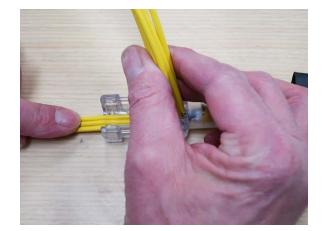
14. Once in place, slowly pull each furcation tube away from the cable sheath to expose approximately 1 inch (2.5 cm) of bare ribbon within the base.
