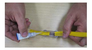
Note: The goal of this step is to securely glue all the tubes together and it is a CRITICAL STEP in the installation process, so don't skimp on the application of the adhesive horizontally and vertically.
