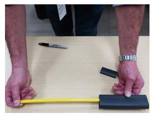
Slide one of the two pieces of 2.5-inch (6.4 cm) heat shrink tubing over the cable stub end.
