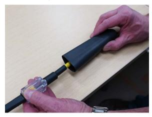
13. Center the 6-inch (15.2 cm) heat shrink tubing between the fused edges of the cable and mesh sleeve.
