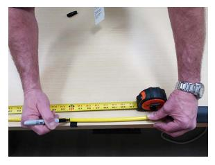
6. Make a ring cut around the cable sheath at the 96-inch (244 cm) mark.
