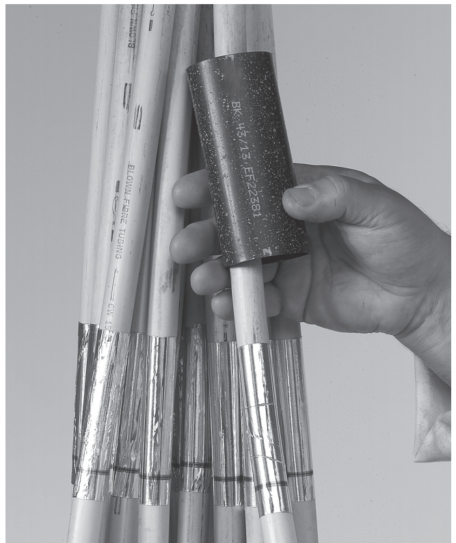
2.5 Slide the heat shrinkable tube over the MDF cable and put it in holding position.
