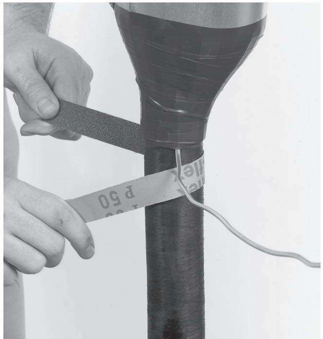
5.2 Abrade the cable jacket with an abrasive strip over ca. 200 mm.
