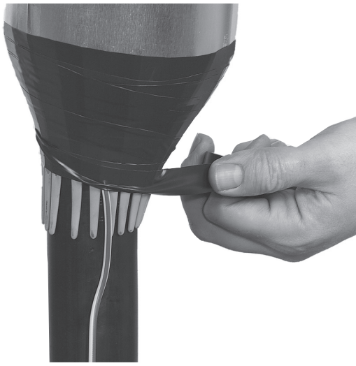
4.3 Tape the crowns of the metal canister down onto the main cable, using PVC tape. Start from the canister body downwards to the main cable with 50% overlap. Tape maximum 5 mm onto the cables.
