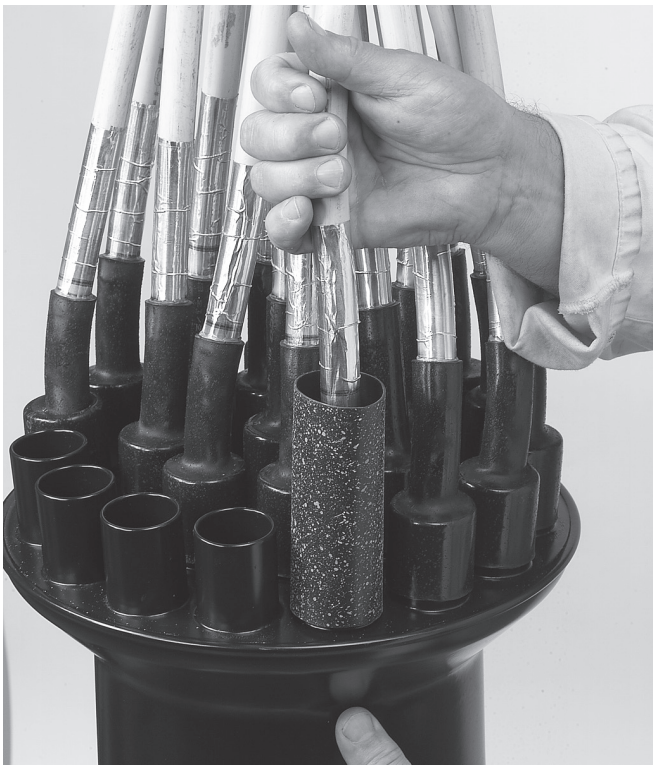
2.7 Position the heat-shrinkable tube over the dedicated port and line up the top of the tube with the base till the top of the tube matches with the blue line of the aluminium cable foil.
