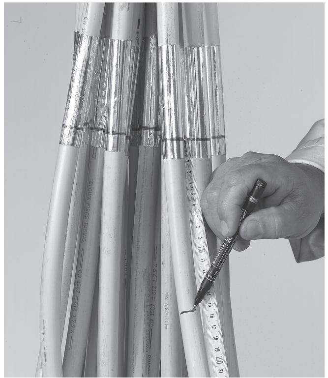
2.4 Measure 150 mm down from the blue line of the aluminum cable foil down to the cable end, mark and remove the MDF cable jacket starting from the mark (jacket to jacket opening should be 740 mm).
