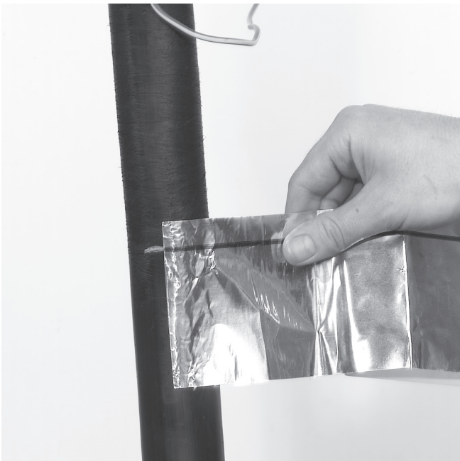
5.4 Wrap cable aluminum foil around the cable jacket, positioning the blue line on the mark. Smooth the aluminum foil with a blunt tool.
