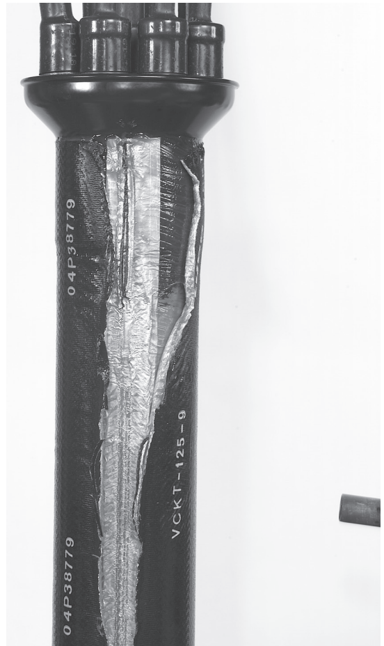
6.3 Heat the sleeve circumferentially until it opens at the channel area.
