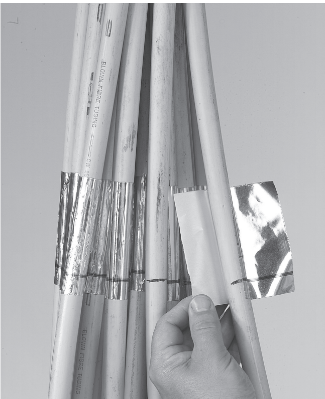
2.3 Apply cable aluminum foil on all MDF cables, matching the blue line with the mark on the cable. Install the foil upwards from the cable mark.
