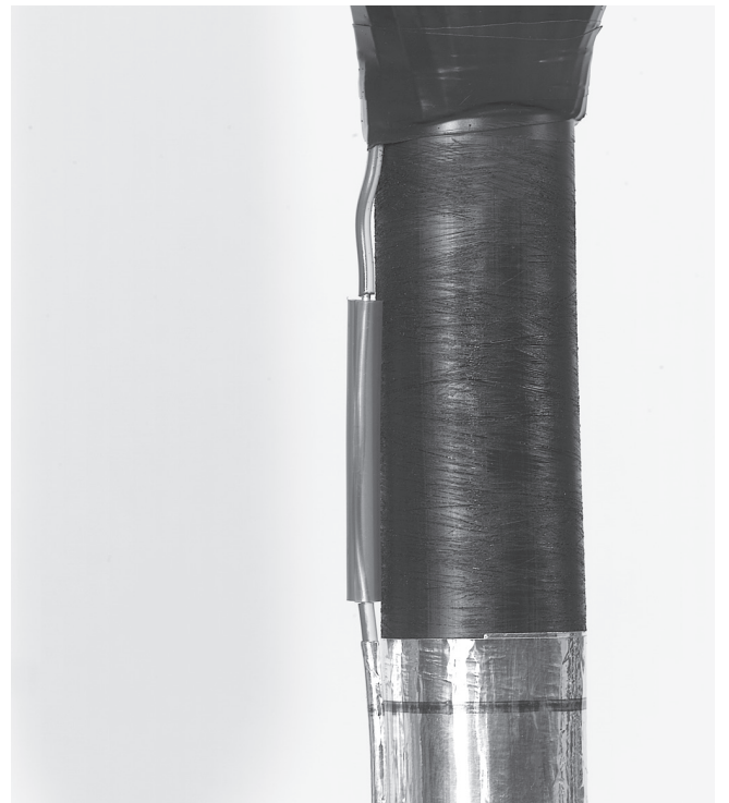
5.7 Install the slitted adhesive tube around the earthing wire over the stripped area of earthing wire.
