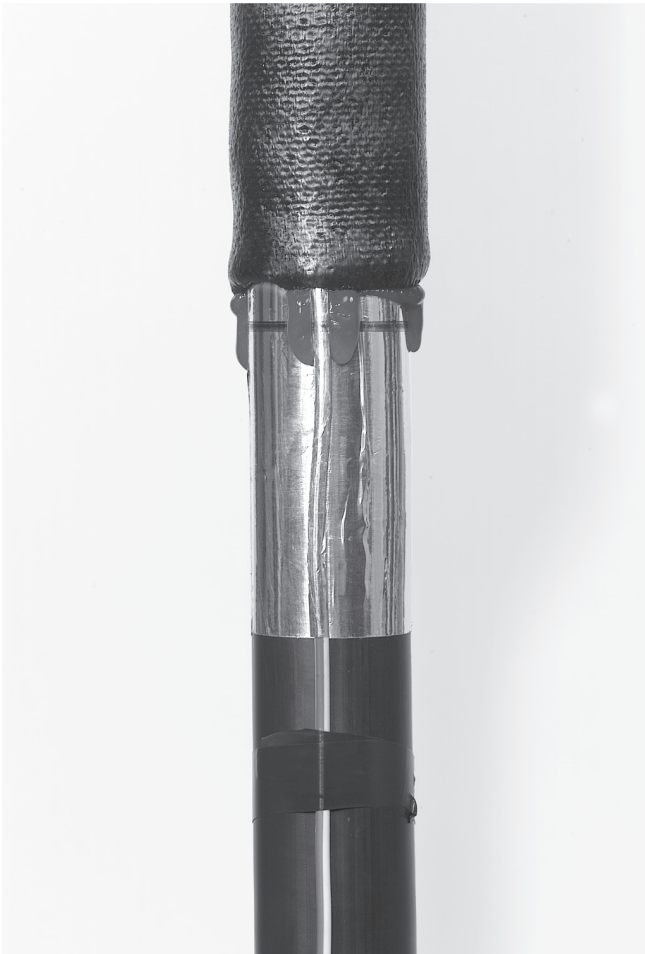
5.14 Apply 10 seconds post heating at the main cable end to ensure a good adhesive flow.
