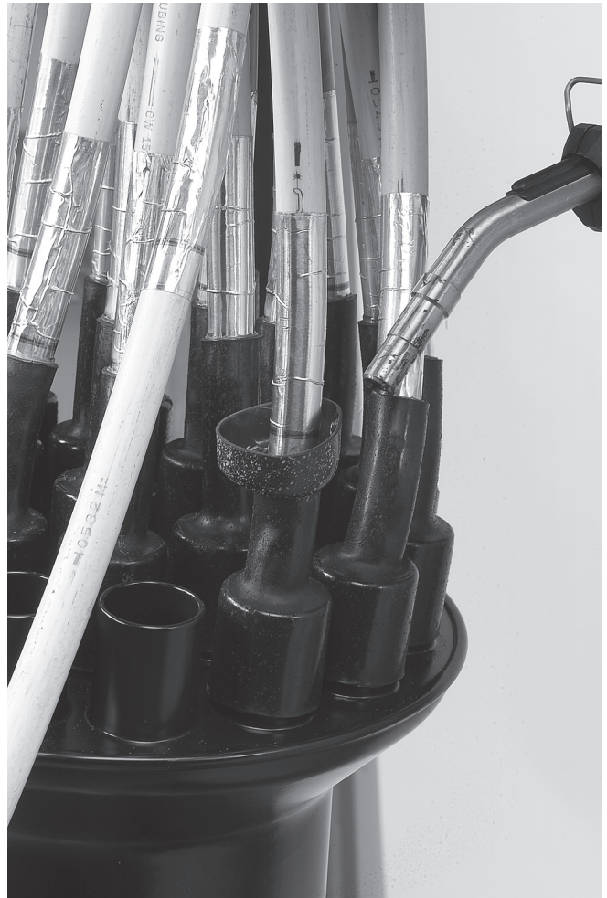
2.8 Shrink the heat-shrinkable tube with an appropriate nozzle (FH-T001-PP14). Start on the metal ports of the distribution outlet in order to fix the tube and continue shrinking up to the MDF cable jacket.
