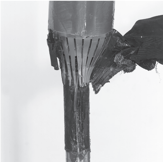
6.6 Remove the PVC tape from the crowns of the canister.
