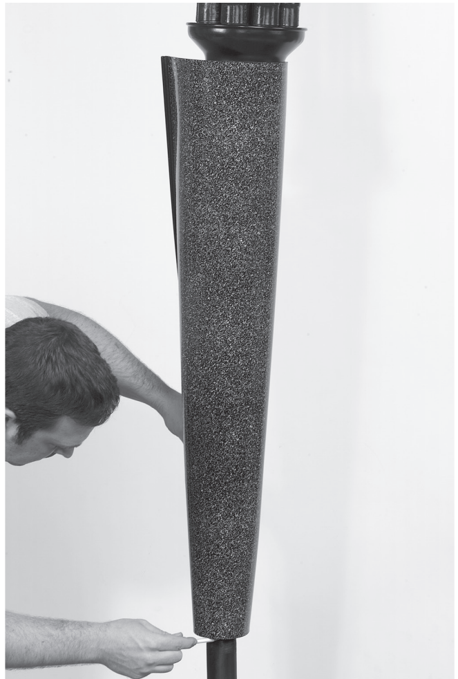
5.3 Center the sleeve over the joint, upper sleeve end positioned over the cylindrical part up to the conical shape of the distribution outlet. Mark the sleeve length on the main cable.
