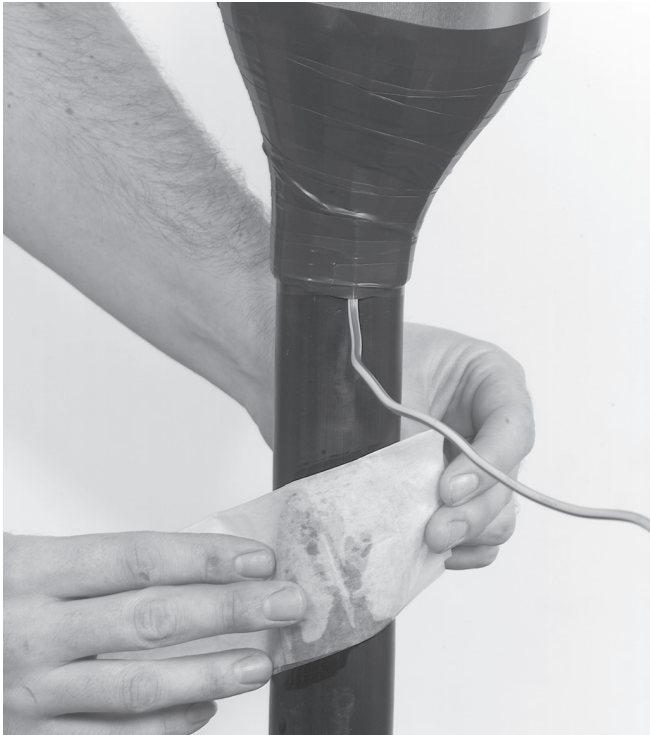
5.1 Clean the main cable jacket with a cleaning tissue over a distance of ca. 250 mm.
