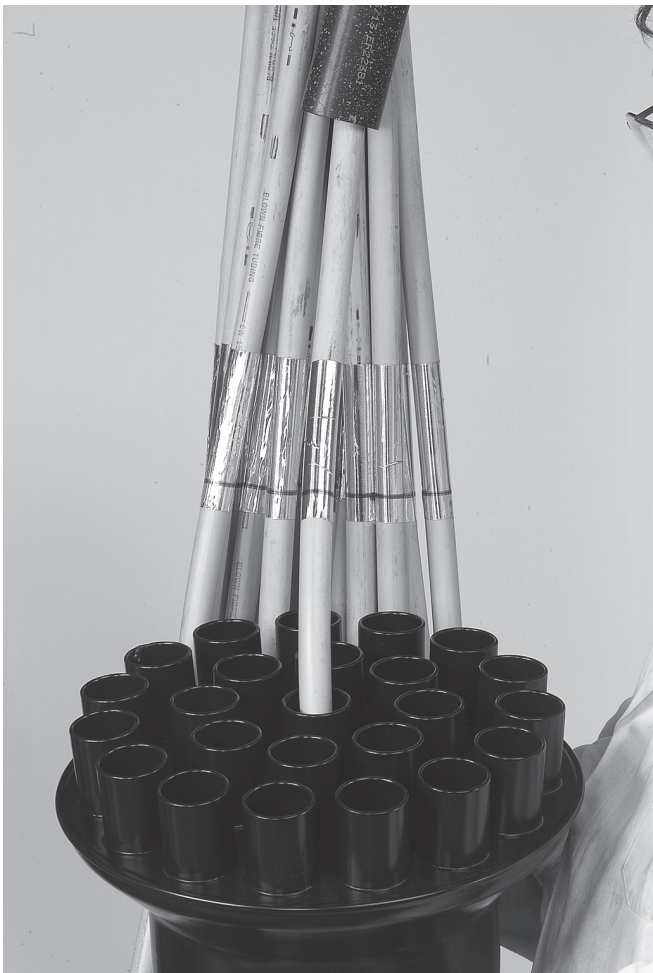
2.6 Insert the MDF cable (one by one) in the dedicated port starting in the middle.
