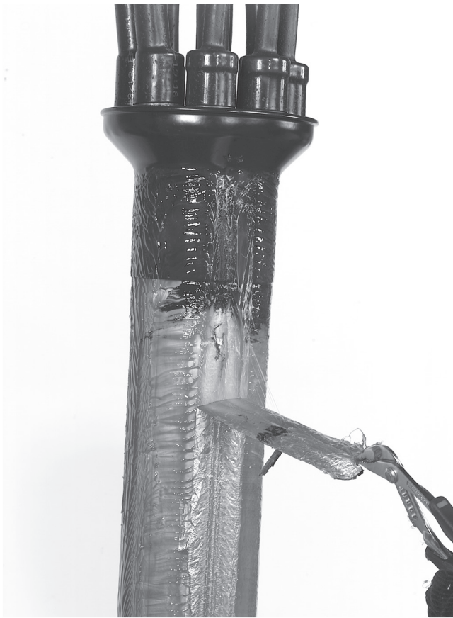
6.5 Remove the flap of the sleeve with a pair of pliers.
