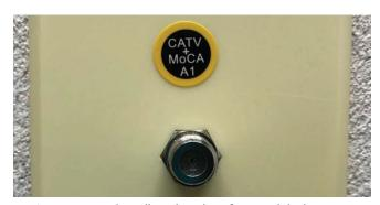
7.2.1 To attach wall outlet identification labels, remove the corresponding circle wall outlet identification label from the sheet and attach it to the wall outlet.
