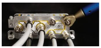
6.2.1 All connections must be torqued to a minimum 20 in-lbs. or according your local system specifications. Use a torque wrench to ensure required torque levels.
