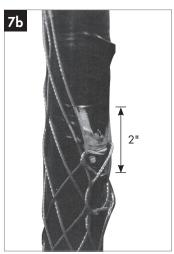
8 Attach the hoist line to the grip as shown in Figure 7. Tie the cable or waveguide leader to the hoist line so that the leader does not dangle. Apply tension slowly to the hoist line to allow the hoisting grip to tighten uniformly on the cable or waveguide.
