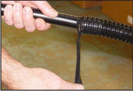
Remove electrical tape from corrugated protection tube
